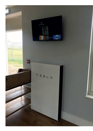
Battery storage gives greater control over how and when you use the energy you generate, allowing you to replace the electricity you buy from the grid with the free electricity your panels are generating. It also provides a back-up in the case of power cuts and ensures the café's fridges and freezers keep running.
